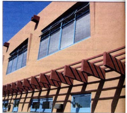
Above and top, architect Beverley Spears' angled shade-structures engineered for the library's west-facing windows
