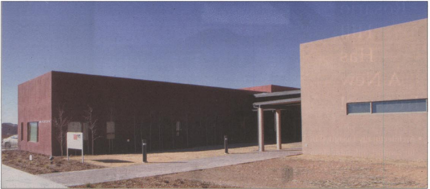
The Santa Fe Rape Crisis Center designed by Spears Architects' James Horn. Below, the local newspaper's new building at One New Mexican Plaza.
